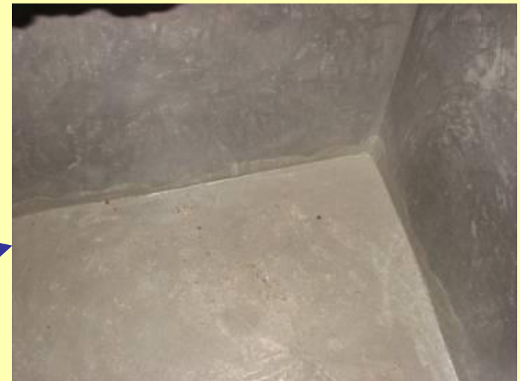
The inside of the tank is repaired and recemented
